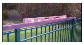
If the installation requires that the fence is level as opposed to following the grade, we find it more effective to use a post from post top to post top and place the level on it rather than on
