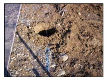
If we're following the pool deck we can use a level at either end and tap the pins down till we reach the right height with the string. Only **two Inches** is allowed between the bottom rail and the <u>finished grade</u>. The string now gives us a point to build our spacers up to.
