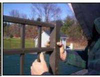
As mentioned previously, loose dirt should never be put back in the hole. This may be a tempting solution if you think you've dug too deep and want to save on concrete. Installation longevity comes from proper post depth so we *purposely* over-dig and drain the posts with a piece of PVC. 1-1/2 inch pipe or electrical conduit is dropped into the post *before* inserting the rail ends. We prefer this method over a 'weep hole' drilled in the post right at grade.
