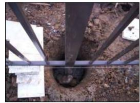
careful about splatter - we remove any before we leave the post. The hole is usually backfilled with dirt; we make a last vertical check with the level and make any final adjustments. We leave the spacers in place and don't disturb this post again. We sometimes even wait till the following day to 'top' the holes; but of course we know the posts are 'perfect' before they're allowed to set overnight.
