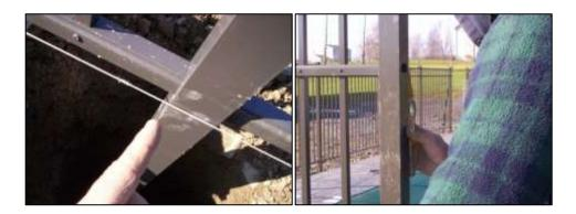
We maintain the 1/16 of an inch gap between the post and the string and constantly check the plumb of the post.
