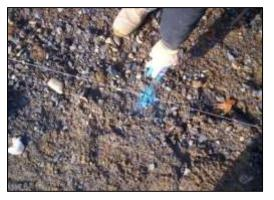
As we place each nail we give it a shot of paint to make it easier to find after we've located all the post centers on each 'run'.
