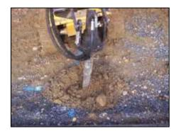
Our machine has side to side as well as front to rear movement of the auger power head. This will help us to get 'around' any large rocks to dislodge them and then return to the correct 'center'.
