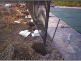
If we 'top' the holes the same day or not, we continue to lay out our spacers and install the sections maintaining the same 1/16 of an inch gap between the post and the string. We move our digging bars from those posts where the concrete has set sufficiently and work toward the corner.
