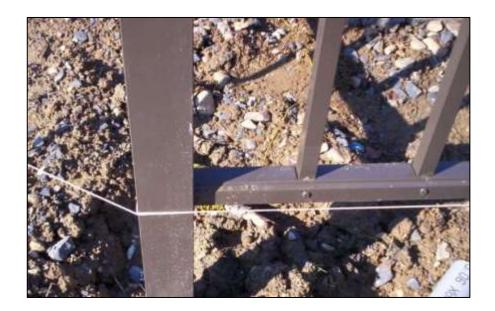
When we're installing we get to a corner, if the position of the string is off just a little for the next run, we move it closer to the post being sure to make a similar adjustment at the other end of the run. Since we've dug a wide enough hole there should be ample room for this change. We then insure the string is as taut as possible (like a piano string), verify height, set our marker stakes between holes and continue with the installation.
