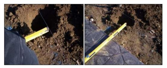
Whether we use a machine to dig or not, the most important part of the hole is the bottom. The bottom should be tamped/packed; we like to use the flat end of the digging bar for this purpose but a 2x4 or 4x4 works equally well. No matter what we use to firm the bottom, the **worst thing that can be done** is to put dirt back in a hole. Packed or not, this can settle in a few years and leave the fence looking like "who did it and ran".
