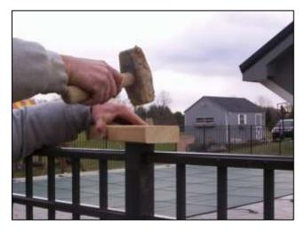
Once we're sure the post is straight; plum and level, and we've given the concrete a chance to harden a bit, we can remove our digging bars and make adjustment to the height paying close attention to the measurement between the bottom rail and the grade. It's better for us to set the post a bit higher at first, but usually no more than ½ inch - we can tap it down before the concrete gets rock hard. The spacers may need to be repositioned but the concrete is firm enough to support the fence. On a
