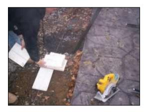
When it's time to install the section we lay out 'spacers' to support the bottom rail and keep the correct clearance from the grade. We use pieces of vinyl fence pickets close to or right at the post. 2x4's or 1x4's work just the same. We keep our eye on where the post is at on the string. Even the best installers can mistakenly throw the line off. On level ground, we can sometimes get 3 or 4 sections ready to be poured at one time.
