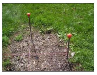
Ideally, a corner is located at the end of a full section. When we set up the corner, we allow for the fact that nails are set at 'centers'. It is best to use 2 stakes at each corner and place them far enough away from the location of the hole so they will not interfere with the positioning of digging equipment or wheelbarrows. We try not to move them once they have been properly placed. However, we are able to adjust the string to the edge of the corner post when it's time to set the
