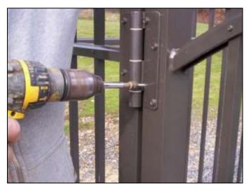
We are extremely careful when using a power tool to install any screws. Overtightening will snap off the head of the screw. After the screw cuts the hole, we 'bump' the trigger till the head gets close sometimes stopping to adjust the clutch or finishing by turning the chuck manually. There are few things more frustrating than snapping the head off the last screw and having to take everything apart to remove it.
