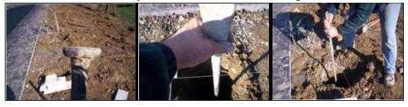
We find it helpful to place a stake at the string line between every hole as a marker to insure a straight run. You might be surprised at how quickly the string, and with it, the fence can wander. The line should remain taut as the fence is set. Marker stakes are removed as we work our way down the line.
