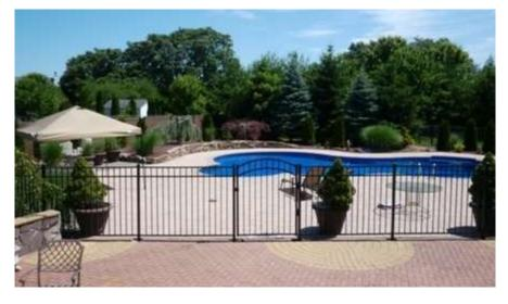
Two fences are recommended for pool safety: a perimeter fence and a fence between the house and the pool. ALL fences should be built at least 48" above grade, measured on the side of the barrier that faces away from the pool, with a maximum clearance of 4" between the bottom of the fence and the ground. No young child should be able to go under, climb over, or go through a fence with these specifications.
