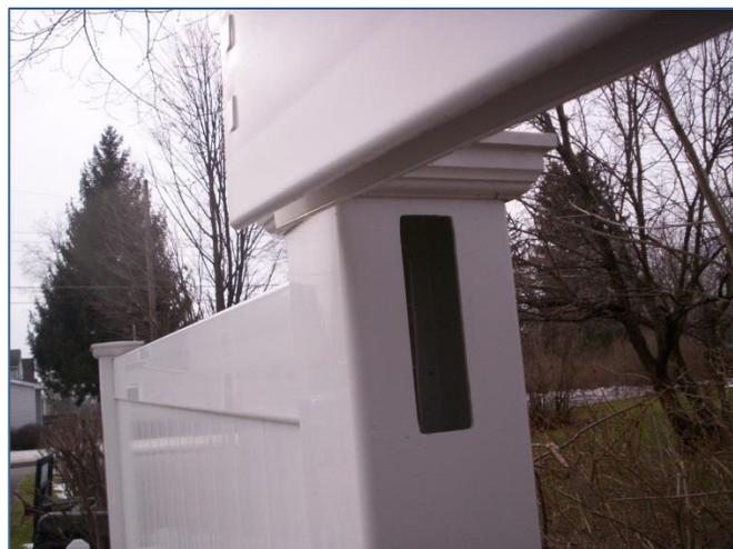
Pickets will now be moved into position in a similar manner - sliding them in from the free end of the top rail which can be pulled toward the installer to facilitate the process. The free hand can be used to steady the top rail and prevent it from moving enough to allow the pickets to fall out.
