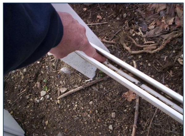
Take the replacement rail and slide it into the hole of one of the posts on the section that is being repaired, push it in till the notches are inside the post and the rail will not pull free. Then set the other rail end on the top of the adjacent post as shown below.
