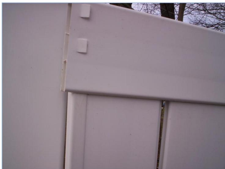
The picket may need to be 'tapped' or wiggled to mate the tongue and the groove over the length of the picket. The top rail is then slid into the opposite post far enough to allow the end of it to be positioned at the routed hole in the post. The rail is slid into the hole far enough for the vinyl tabs to lock in place.
