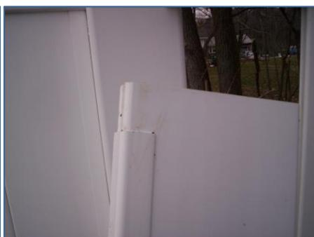
Holding the picket on a slight angle, slide the bottom of the picket into the slot of the lower rail while being mindful that its bottom edge on the opposite side may get caught on the lip of the rail. Very often the picket can be manipulated into place by wiggling it and applying downward pressure. If this does not work, a free hand can be placed between the pickets and used to force the bottom toward the installer while pushing down with the other hand.
