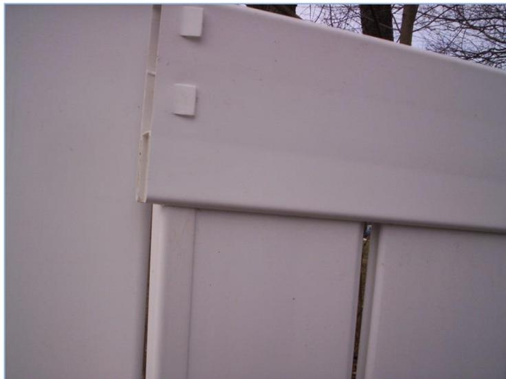
The picket may need to be 'tapped' or wiggled to mate the tongue and the groove over the length of the picket. The top rail is then slid into the opposite post far enough to allow the loose end of it to be positioned at the routed hole in the post. The rail is slid into the hole far enough for the vinyl tabs to lock in place.
