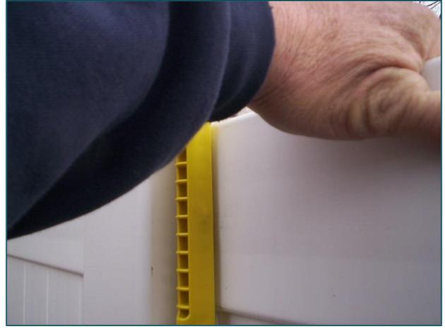
Once the rail has been removed any pickets left in place will drop if they didn't do so previously. It is not necessary to remove both ends of the rail if the tabs have not been damaged. The free end of the rail can be set on the top of the adjacent post as shown below.
