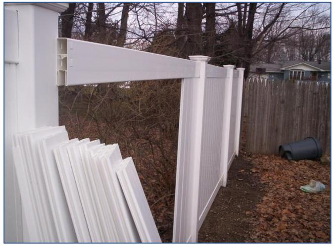
Continue to install pickets in this manner until the last picket to be installed is reached. The second picket with 'U' channel will now be used to finish the 'field'; this part can be a little tricky and will require some patience.
