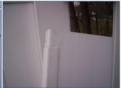
Holding the picket on a slight angle (left/right), slide the bottom of the picket into the slot of the lower rail while being mindful that its bottom edge on the opposite side may get caught on the lip of the rail. Very often the picket can be manipulated into place by wiggling it and applying downward pressure. If this does not work, a free hand can be placed between the pickets and used to force the bottom toward the installer while pushing down with the other hand.
