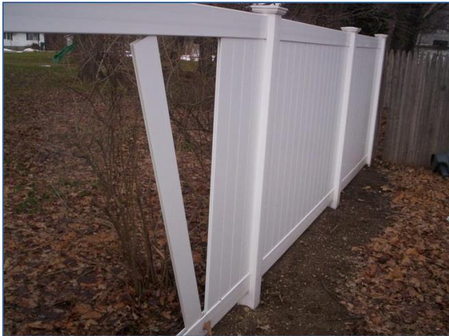
Continue to install more pickets until you reach the point where the space between the rails is too great for the top of the picket to slide into the top rail and remain upright.
