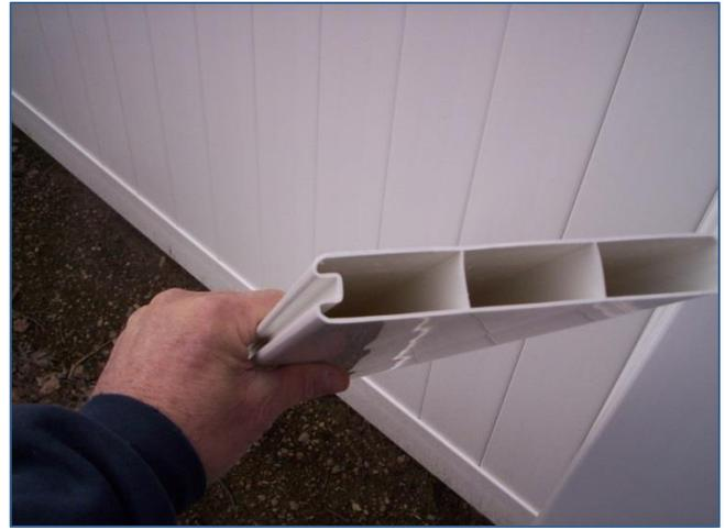
Holding the picket with 'U' channel on it at an angle, place the bottom corner into the slot of the bottom rail, align the top of the picket with the slot in the top rail and move the picket into the vertical position with the 'U' channel flush against the post.
