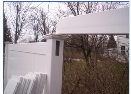
The slot in the bottom rail should be cleaned of any debris so the pickets mate well. Using a rag or paper towel, dirt and grime can be pushed toward the rail opening in the post and be swept into it. The top rail can now be set up to reinstall the pickets.
