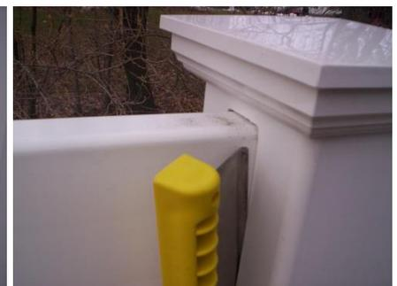
The tool is inserted into the gap between the rail and the post by holding it at the angle that allows the curved end to lay flush on the rail. When fully inserted, the metal will allow the tabs to slide past the inside edge of the post and the rail will come free.
